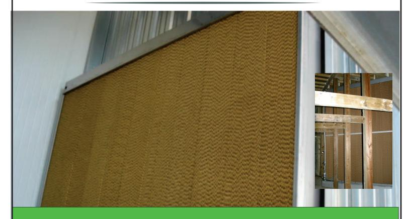
The Humi-Cell is a passive humidifer that allows the air passing through it to be fully saturated. The water holding capacity of the air is the control for the Humi-Cell. Techmark's Humi-Cell is a high quality product and a productive addition to all storage ventilation systems.
